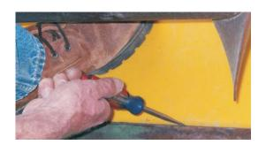
6. With the Poly panel pushed fully to the rear and the rear mounting holes aligned, pry the front edge of the panel behind and under the steel plate at each row with a large screw driver or pry bar.
